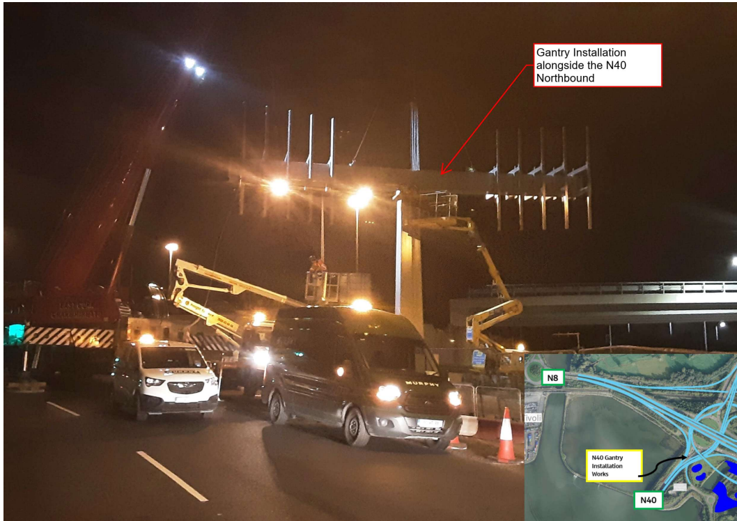
Gantry installation alongside the N40 Northbound.
