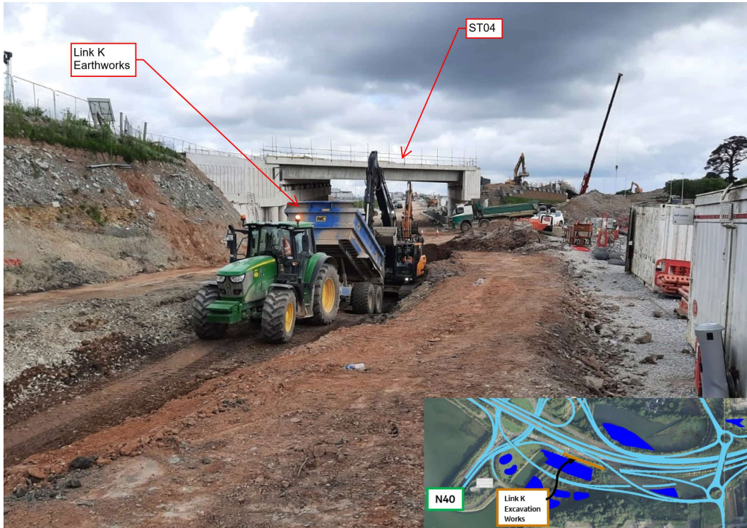
Earthworks ongoing on Link K alongside the N25 Westbound.
