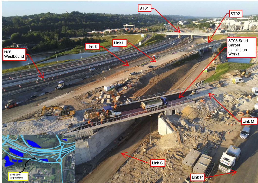
Structure ST03 sand carpet installation works.
