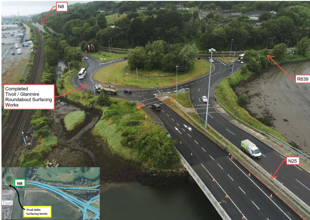
Tivoli Roundabout surfacing works.
