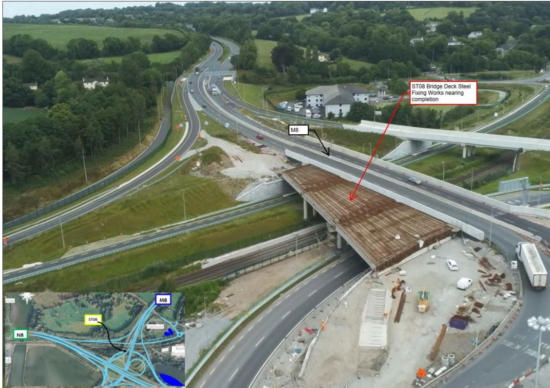
Steel fixing works ongoing at Structure ST08.
