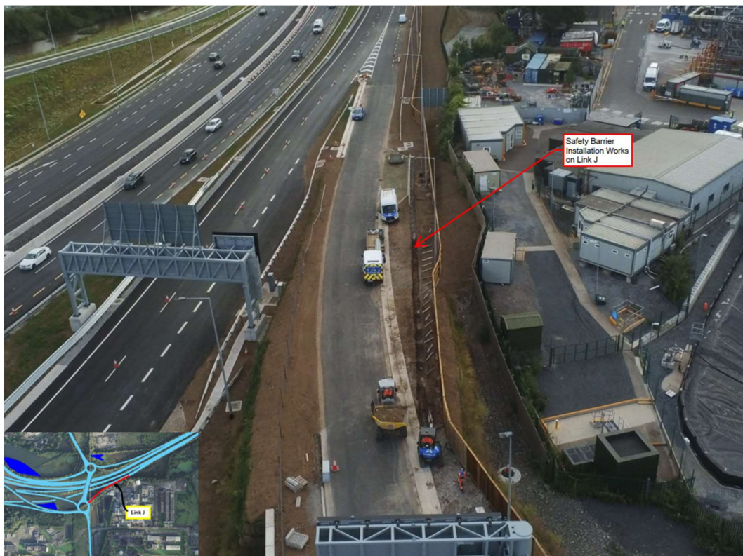
Safety Barrier works at Link J
