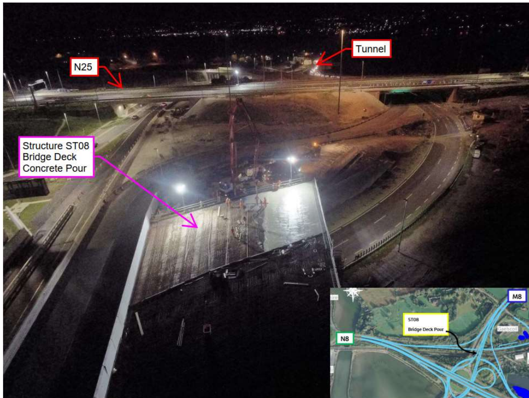
Completion of the bridge deck pour at ST08 ongoing
