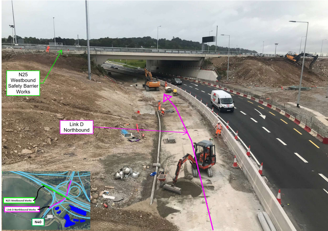
Works ongoing in the vicinity of the old Dunkettle Interchange Roundabout.
