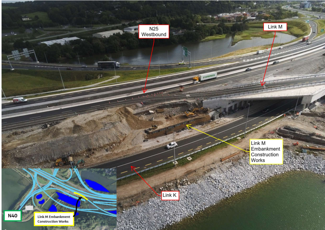
Embankment construction works ongoing alongside the N25 Westbound.
