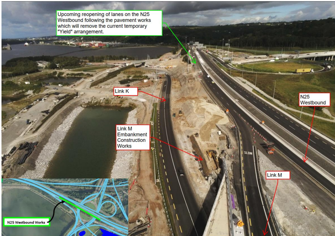
Upcoming pavement works on the N25 westbound.
