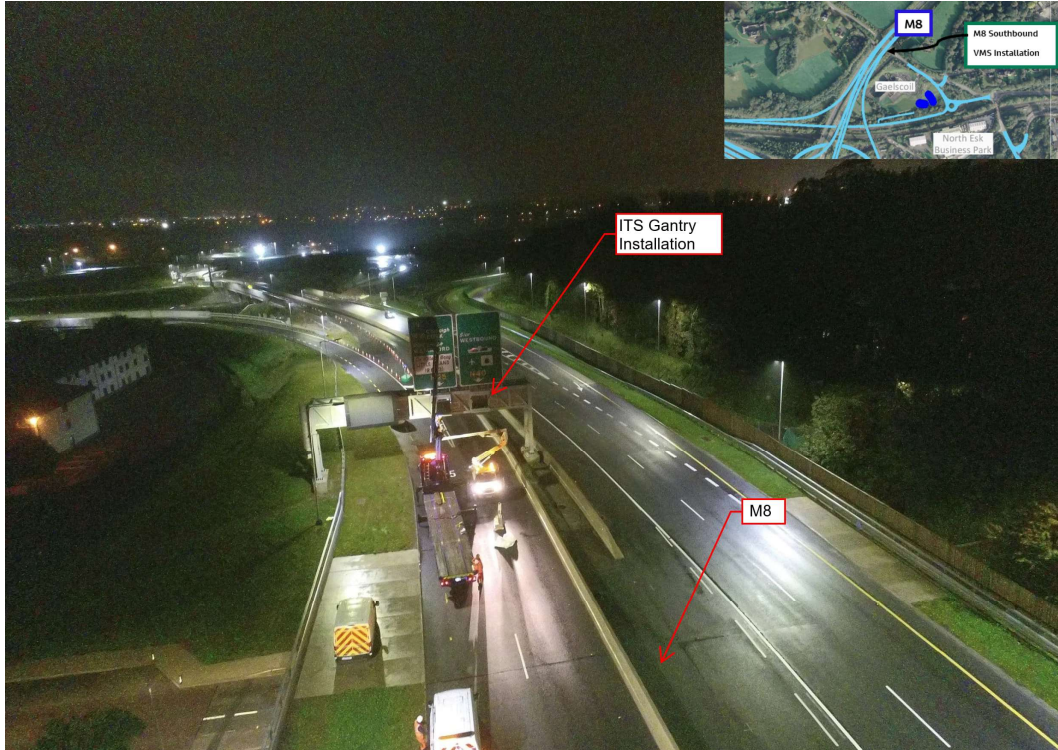
VMS installation works ongoing on the M8 southbound
