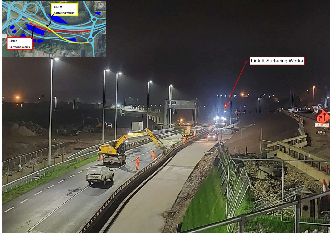
Surfacing works ongoing on Link K alongside the N25 Westbound
