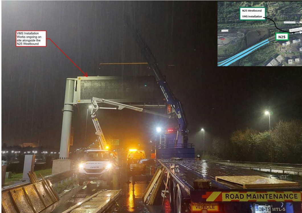
Installation of VMS signs ongoing on the N25 Westbound
