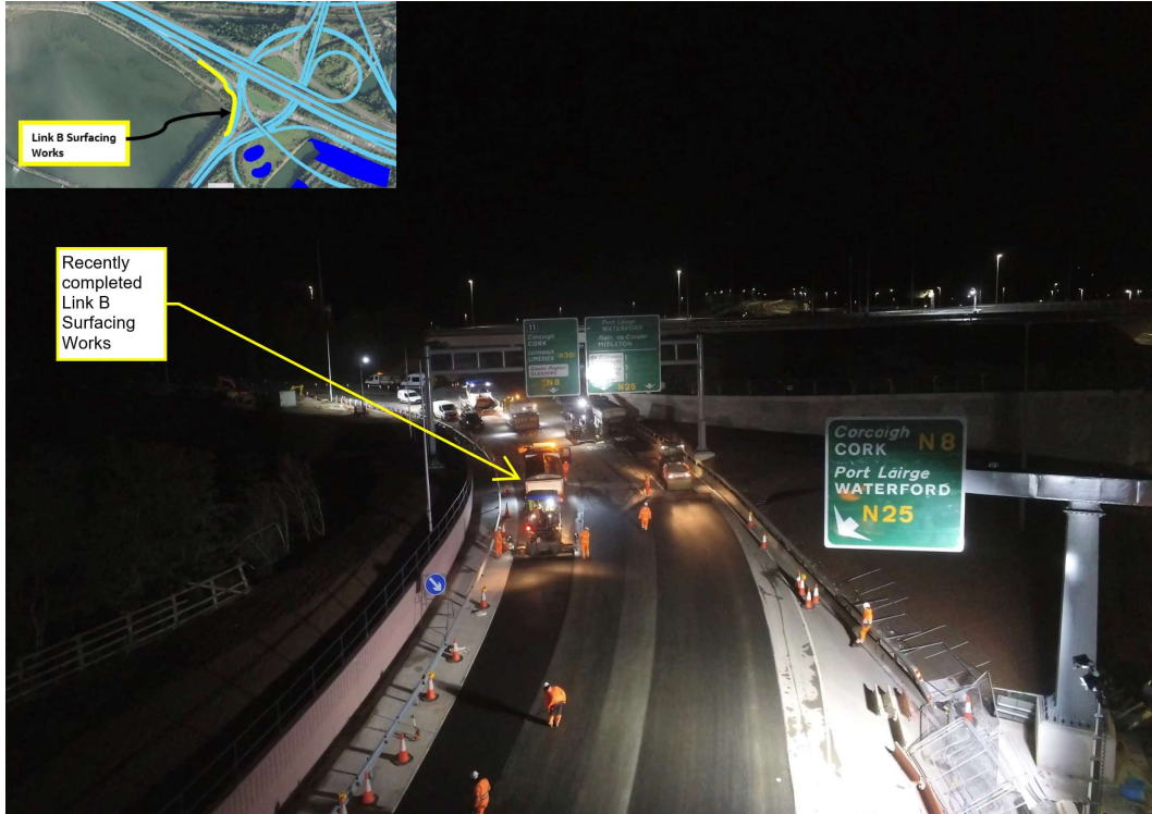
Surfacing works being completed on Link B under night-time working
