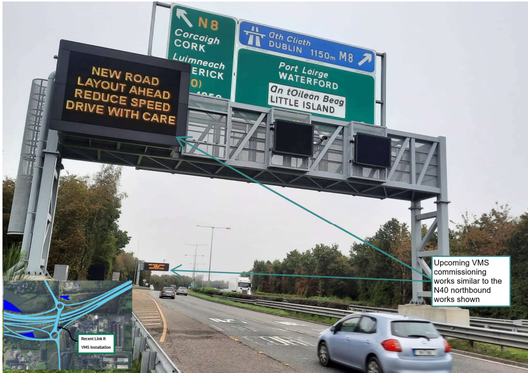
Upcoming VMS commissioning works
