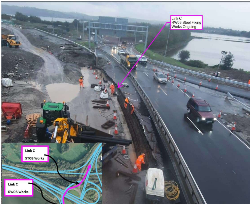
Steel fixing works ongoing at Retaining Wall RW03.
