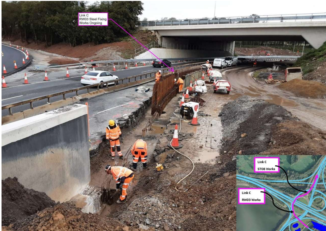
Steel fixing works being progressed at Retaining Wall RW03
