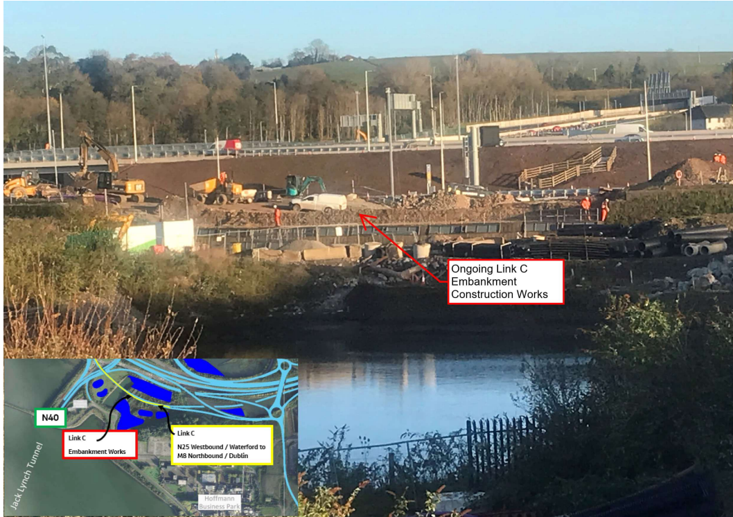
Earthworks ongoing on site for the completion of the Link C embankment
