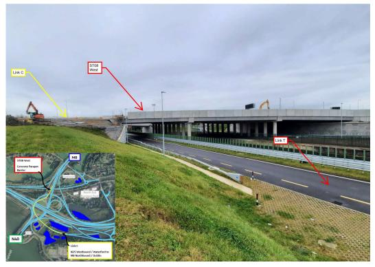
Concrete parapets installed at Link T for ST08 (West)
