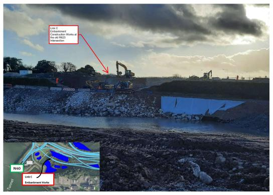
Embankment Construction Works ongoing for Link C at the intersection with the old R623 road
