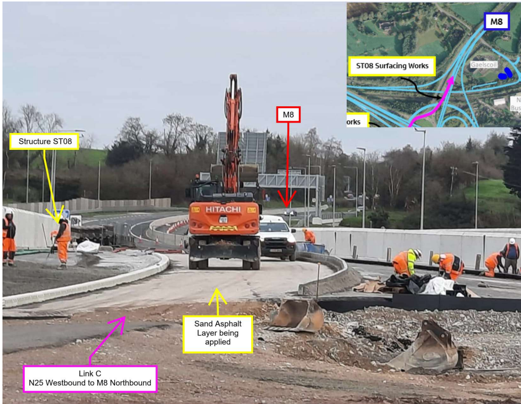
Surfacing works at Structure ST08 (West) on Link C
