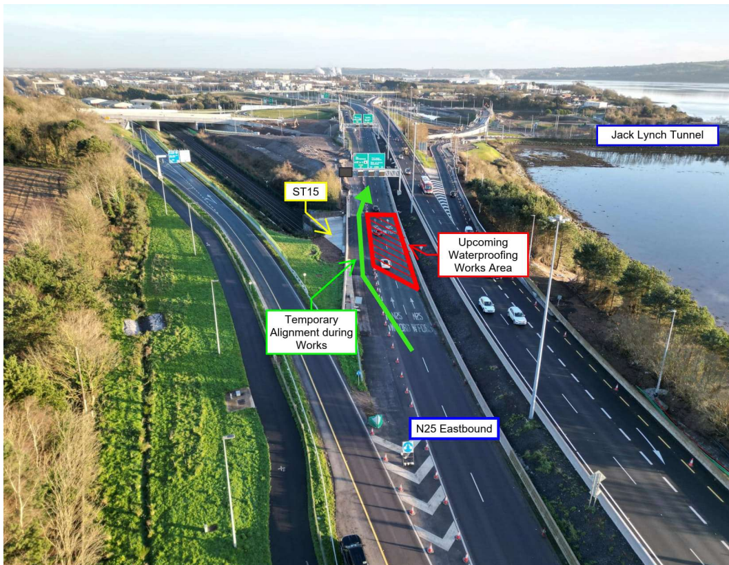
Area highlighted shows the extent of bridge deck waterproofing required
