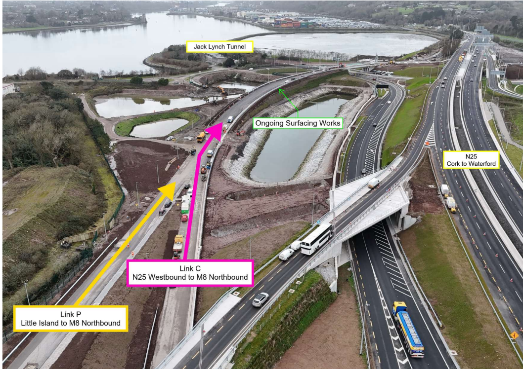
Ongoing works at Link C and Link P
